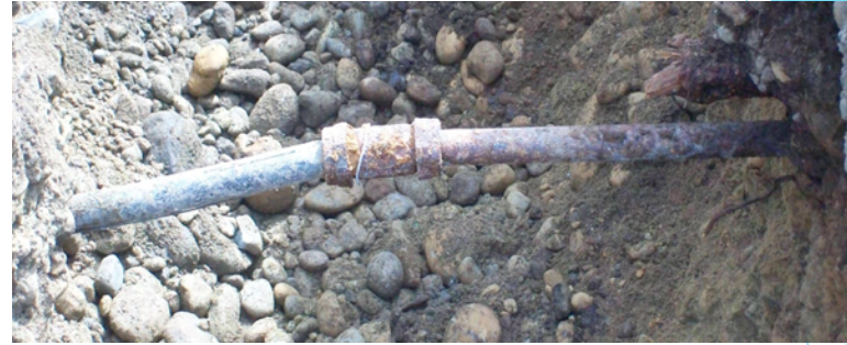
Repaired sewer service project
