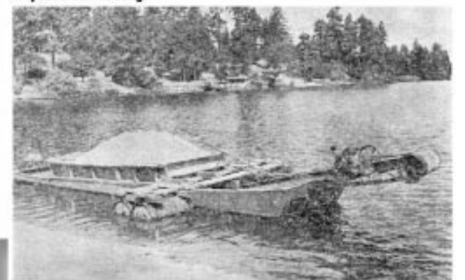
Long a headache for Steilacoom Lake residents is the problem of creating smooth, clean beaches on shorelines that once were mere dirt-covered benches above a swamp or creek bed. Steilacoom Lake, until about the time of World War I, was much smaller lake than it is today, and was mostly a swamp, with a pair of creeks flowing down the middle. To solve the problem of creating clean beaches, Ernie Hedlund, local entrepreneur & Sand & Gravel retailer, built a self-propelled gravel barge. A small gas engine on the barge's deck propels the barge. Thus a customer can have a beach on a few hours.
